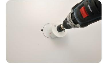
**3.10** Use Ø 79-83 mm hole saw at an angle to scribe cutting radius on the other side.
