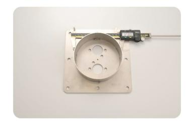
**3.19** Use a deburring tool to remove sharp edges. Check turret sleeves into the drilled hole. Depending on the substrate drilled the mounting floor plate may be a snug fit. Don't insert turret until heater mounted as it may be difficult to remove.
