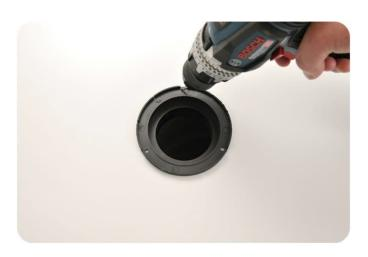
Mount outlet nut. Fastens not supplied in kit due to installation variances. Pictured is a 75 mm nut.
